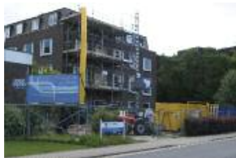
The Stephen Perse Sixth Form College under refurbishment 2007
