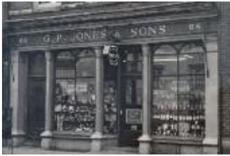
68 Trumpington Street (first premises)
